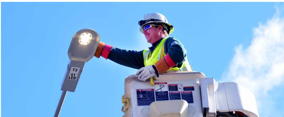
Smart lighting helps customers reduce their energy consumption.
