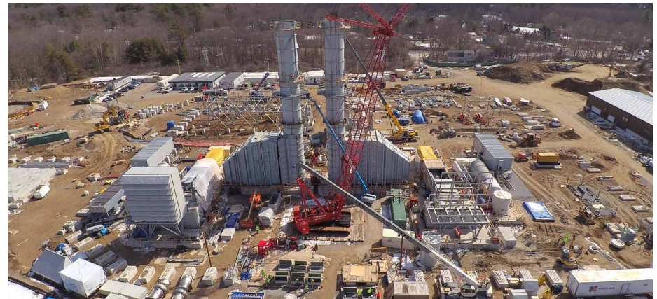
State-of-the-art peaking plant under construction at Medway.
