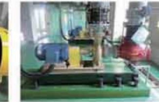
IAC replaced 12 cooling pumps, 3 booster pumps, and grey water pumps in the utility building B and the office building with highly efficient pumps, which is expected to reduce 101.7tCO<sub>2</sub> in GHG emissions per year.
